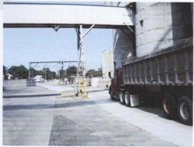
Yoder Concrete completed the asphalt pavement removal, including several old foundations, and the concrete placement in three days. The existing asphalt pavement was removed and replaced with an 8 inch thick concrete steel reinforced drive. The existing stone base was re-compacted in place.
